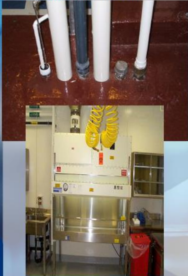
Sealed pipe penetrations
