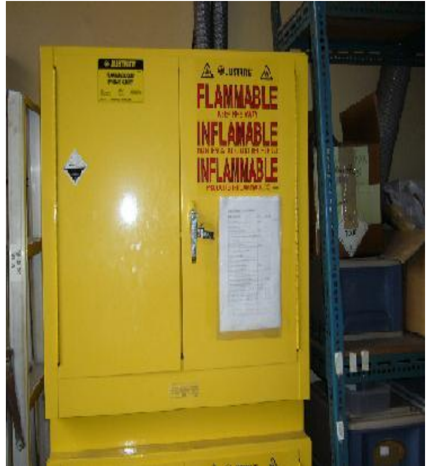
Fire and explosion safety cabinet
