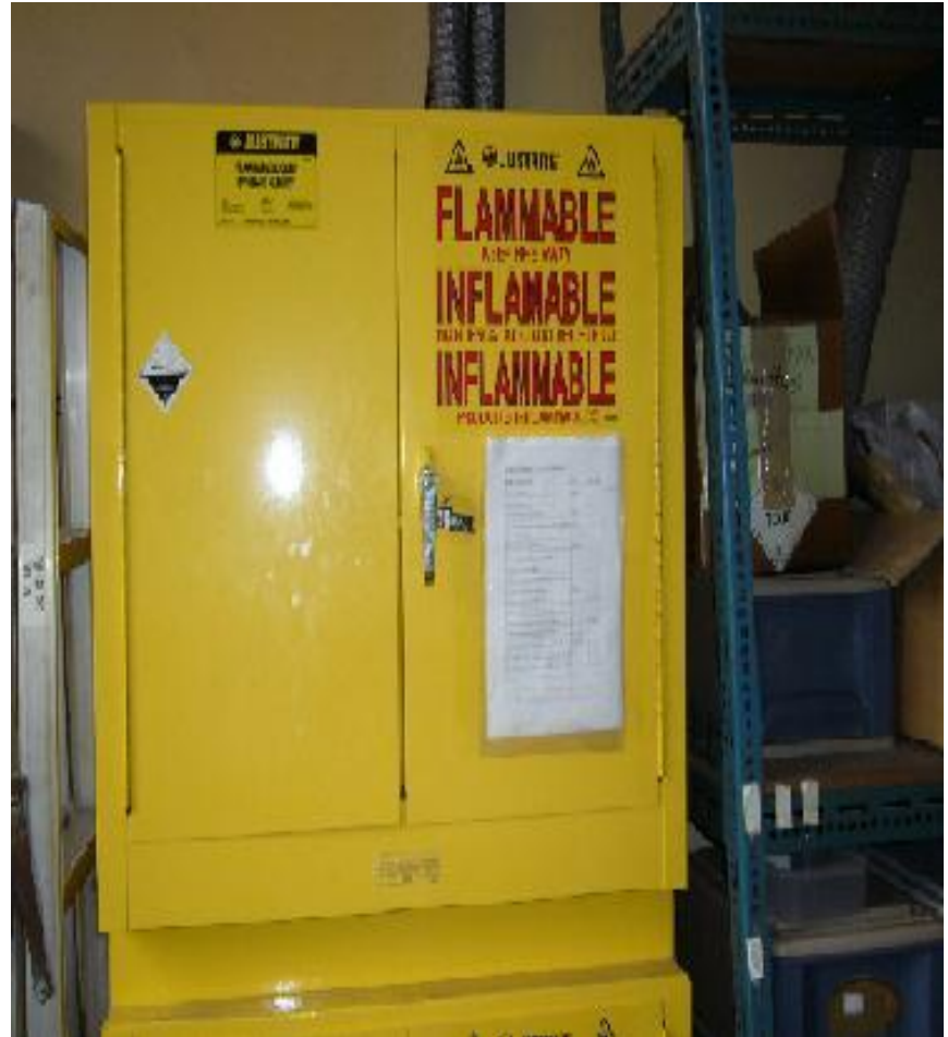
Fire and explosion safety cabinet
