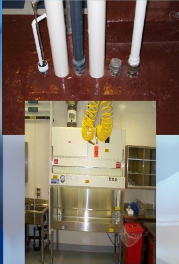
Sealed pipe penetrations
