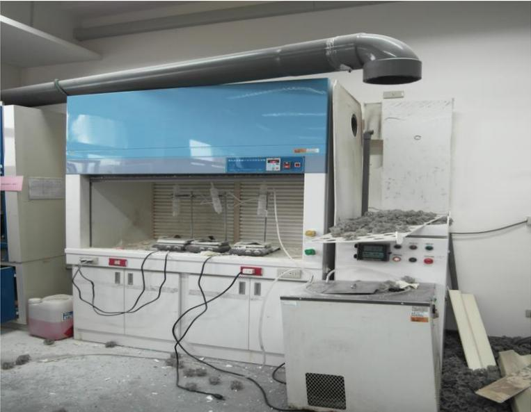
A photograph of a laboratory fume hood. The blue glass front panel is broken and hanging off. The white ductwork above the hood is also damaged and partially detached. The hood is cluttered with various pieces of equipment and debris on the work surface.                                     | <p>圖 2 為事故現場排煙櫃玻璃、導管及水洗式廢氣清淨裝置本體已經破損、脫落。</p>                                                                                     |
